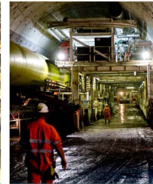
INVESTMENT & FACILITY MANAGEMENT DIVISION
